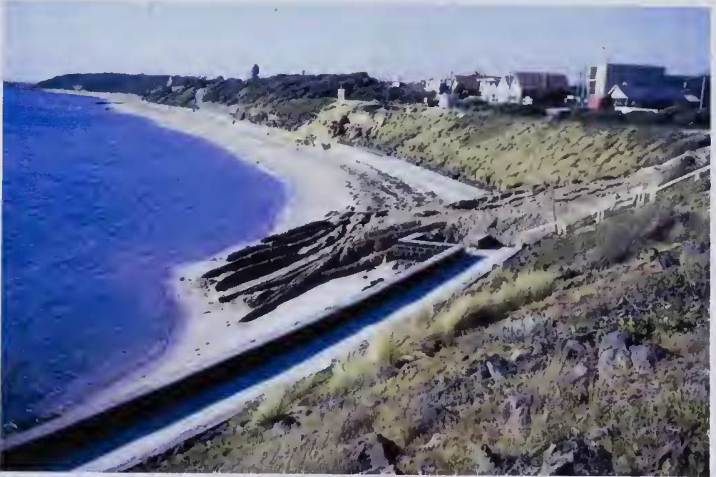
Fig. 8. Sand dumped on the shore near Quiet Corner, December 1969. It drifted away to the north during the next four months, and did not provide winter protection for the sea wall.
